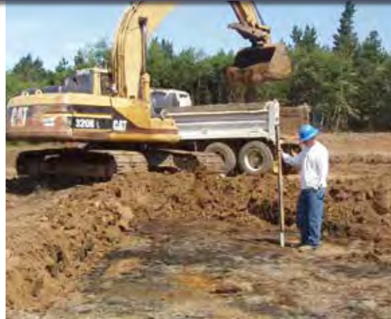
Figure 107. Using rod and laser level to check elevation levels during grading.
