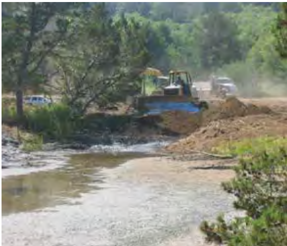
Figure 117. Filling interior ponds.
