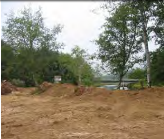
Figure 114. The dike along the Salmon River was cleared of vegetation, but is still present in this photo. The U.S. Highway 101 bridge over the Salmon River is in the background and the tide gate house is still standing.
