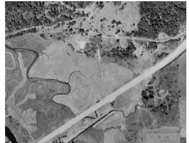
Figure 82. 1961 aerial photo of U.S. Highway 101 under construction. Salmon Creek has been relocated into newly constructed ditches.
