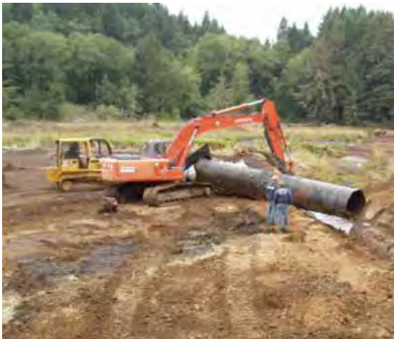
Figure 109. Removing the culvert at the tide gate.
