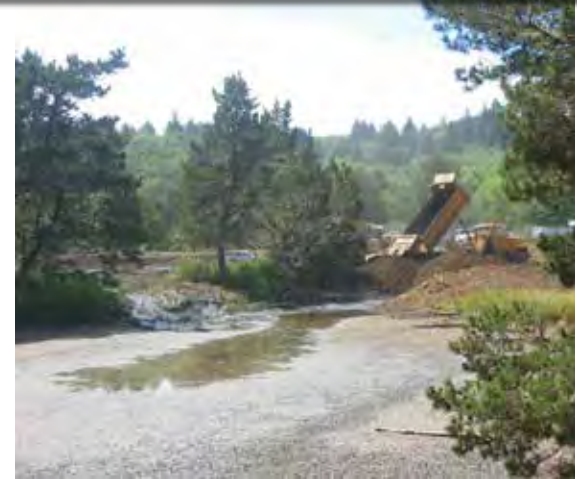
Figure 116. Filling interior ponds.
