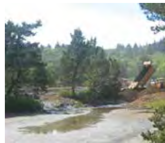
Figure 46. Filling interior ponds.
