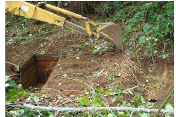
Figure 24. Decommissioning failed septic tank.
