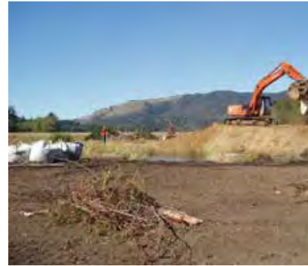
Figure 14. Removal of the final portion of dike that surrounded the development.
