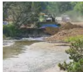
Figure 47. Filling interior ponds.
