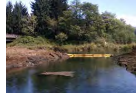
Figure 52. The morning after the tide gate was removed, August 25, 2011.
