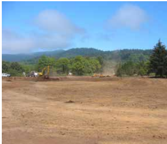
Figure 118. Removing fill from the restored marsh surface, work in progress.
