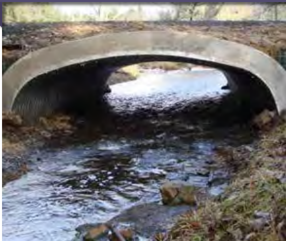
Figure 101. New Rowdy Creek culvert, built in 2008.
