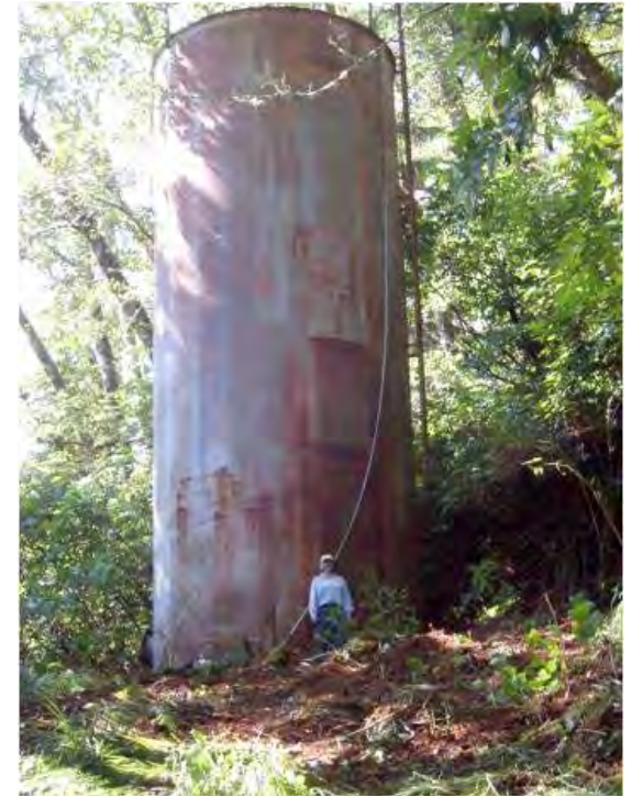
Figure 23. 35 foot water tank for gravity-fed drinking water system.
