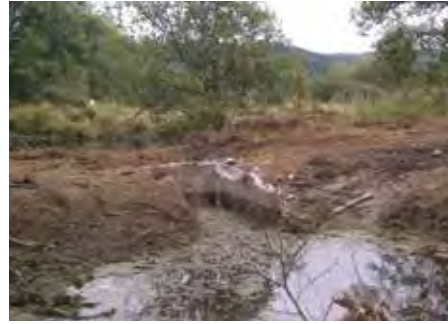
Figure 50. August 22, 2011 site prep for tide gate removal.
